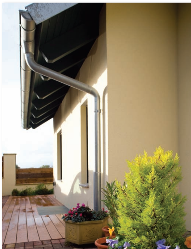
THE UPSHONS SELECTED GALVANISED GUTTERING. THE GRATING IN THE DECKING IS OVER THE LIGHT TUNNELS TO THE BASEMENT
