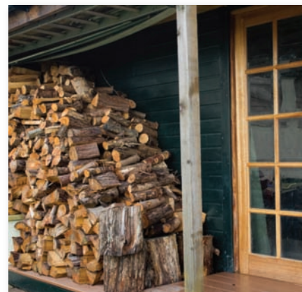
THE STOCK OF LOGS MAY LAST A WHILE – SO FAR, THE NEAR-PASSIVHAUS HOME HASN'T NEEDED HEATING
