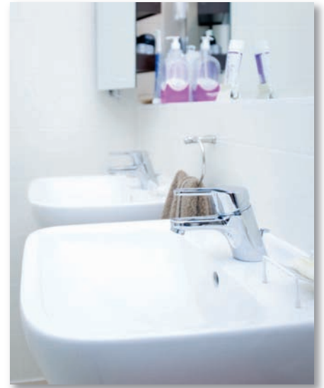
ALL SANITARYWARE WAS SELECTED AT HANSE HAUS BEFORE THE BUILD BEGAN
